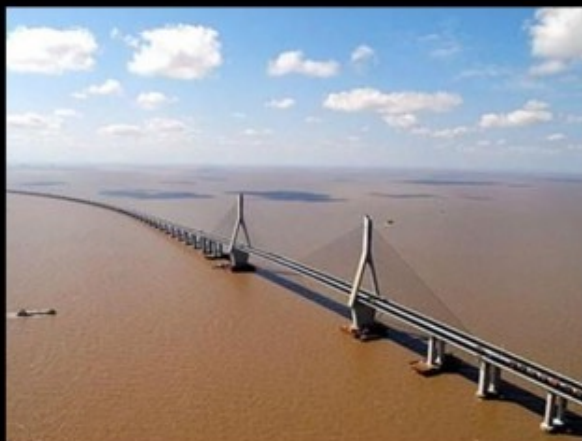
Hangzhou Bay Bridge
