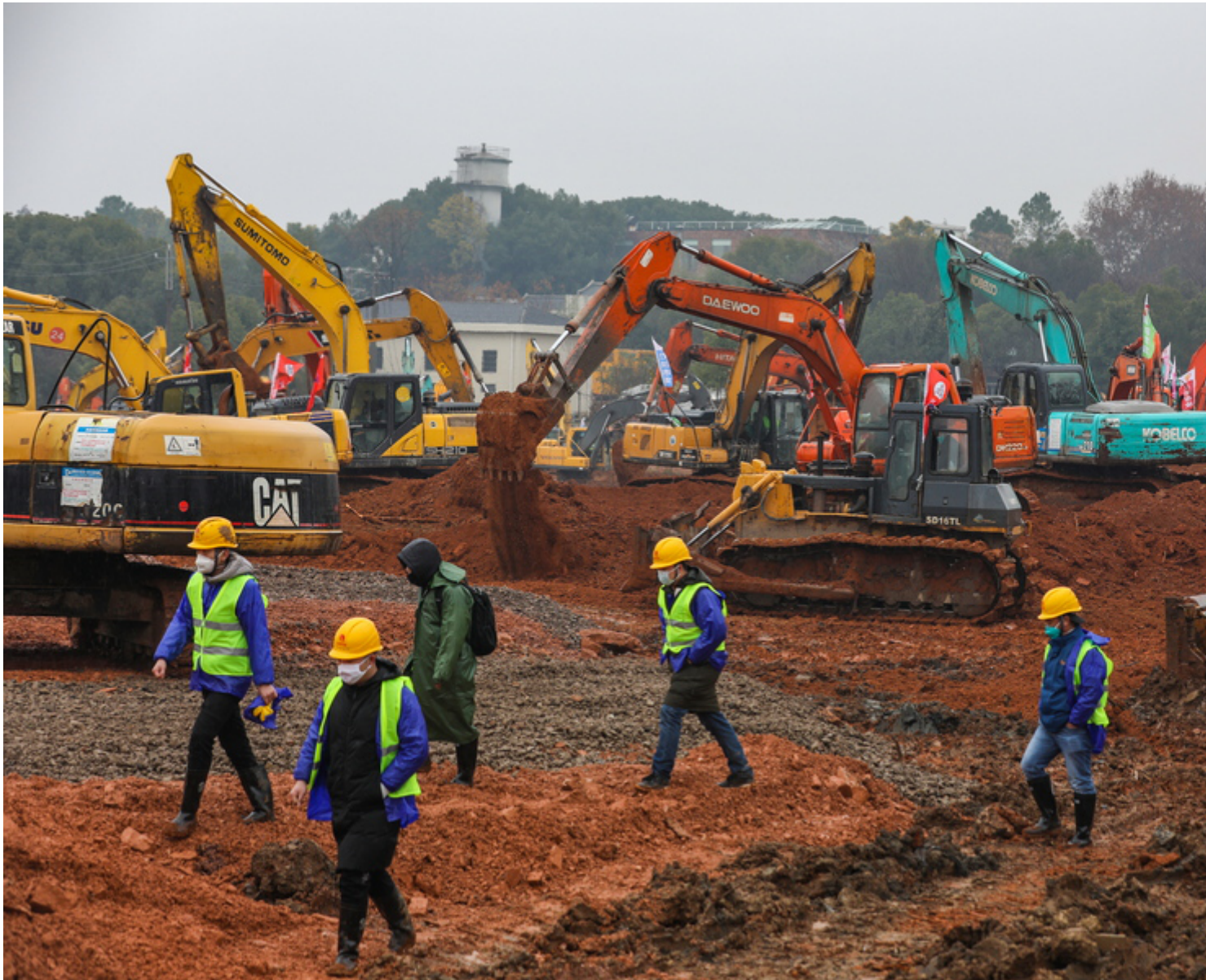
epa08157643 People work at the construction site of a field hospital in Wuhan, Hubei province, China, 24 January 2020. The hospital is expected to be completed by 03 February 2020 to cope with the increasing number of people affected by the coronavirus. The coronavirus has so far claimed 25 lives and infected more than 800 others, according to media reports. The virus has spread to Thailand, South Korea, Japan, Singapore and Taiwan. EPA/YUAN ZHENG CHINA OUT
