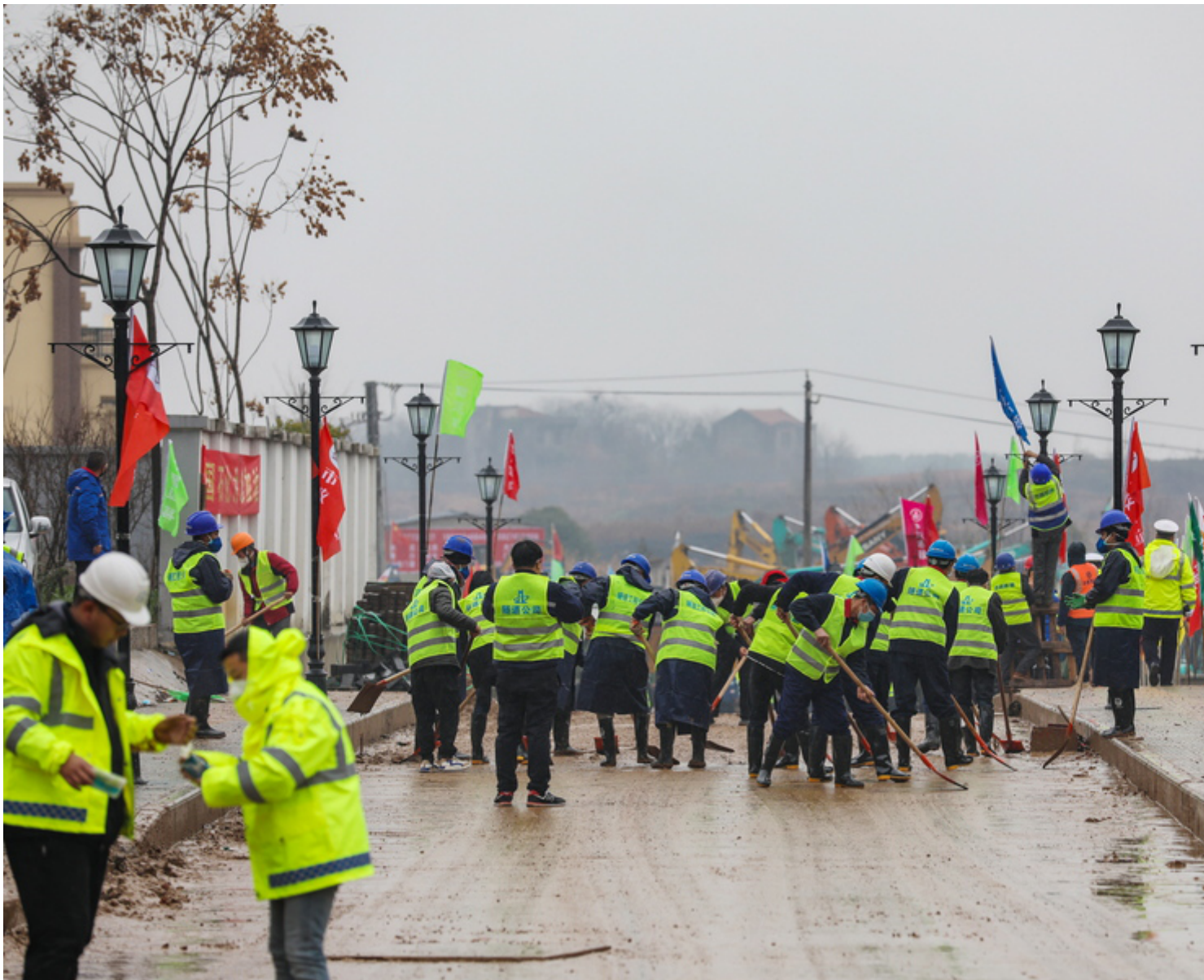
epa08157640 People work at the construction site of a field hospital in Wuhan, Hubei province, China, 24 January 2020. The hospital is expected to be completed by 03 February 2020 to cope with the increasing number of people affected by the coronavirus. The coronavirus has so far claimed 25 lives and infected more than 800 others, according to media reports. The virus has spread to Thailand, South Korea, Japan, Singapore and Taiwan. EPA/YUAN ZHENG CHINA OUT
