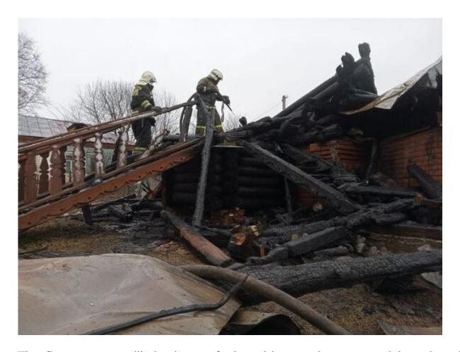
The fire was most likely due to faulty wiring, perhaps caused by mice chewing through the wires.
